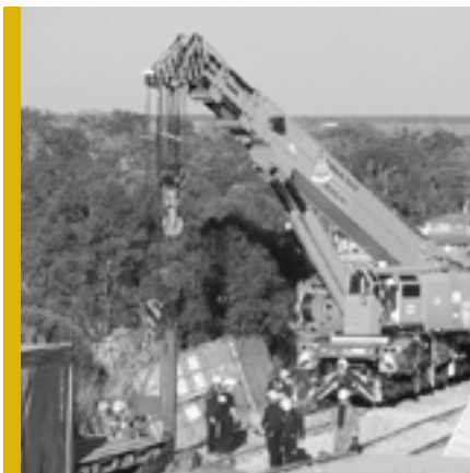
Firefighters working with State Rail following a train derailment.
