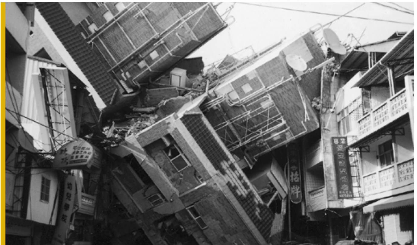
A scene from the Taiwan earthquake captured by Station Officer Wayne Staples.
