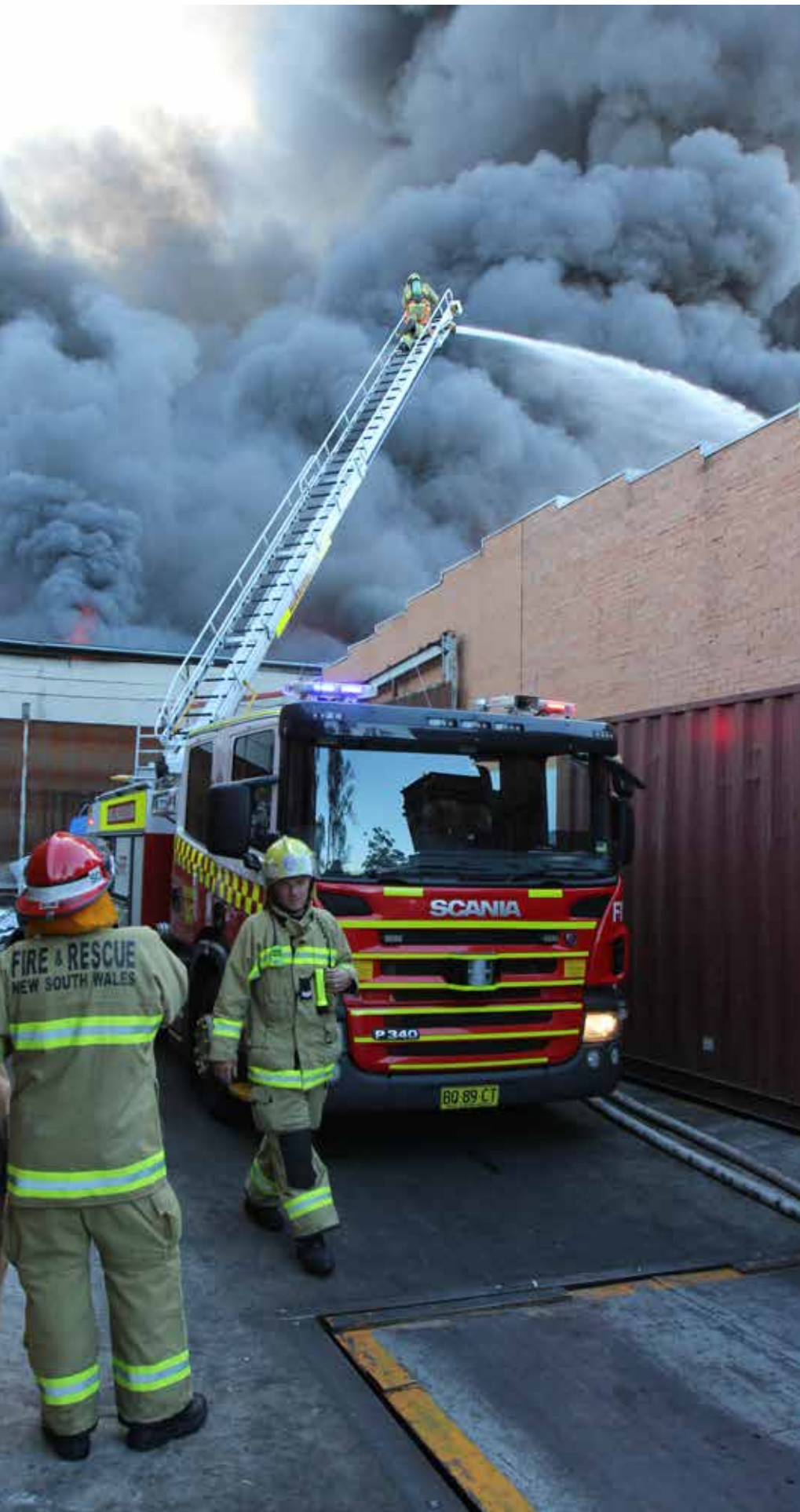
From Sector Charlie, Aerial Pumper 47 positioned outside the collapse zone, provides protection to Sector Charlie exposures.
