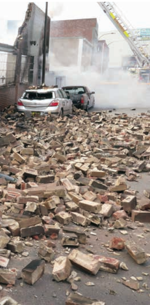
This view shows the projection of bricks to the opposite side of the lane that occurred following collapse of the parapet wall.
