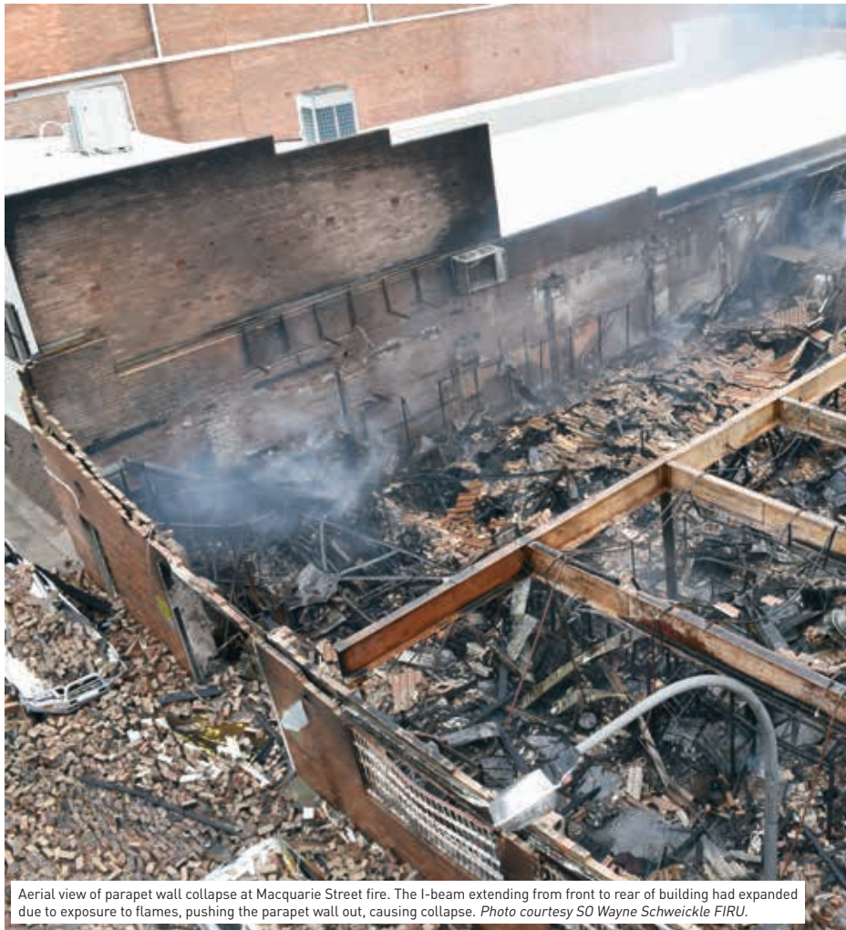
The I-beam is visible in the centre of the photograph sitting on the wall. This I-beam expanded and pushed the parapet wall out resulting in collapse.
