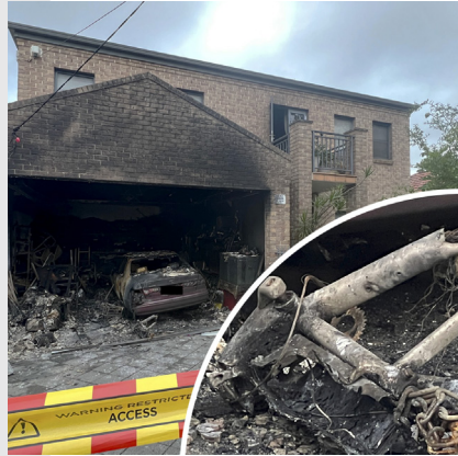
The result of a faulty lithium-ion battery on an E-bike, causing a fire, which had badly damaged the home.
